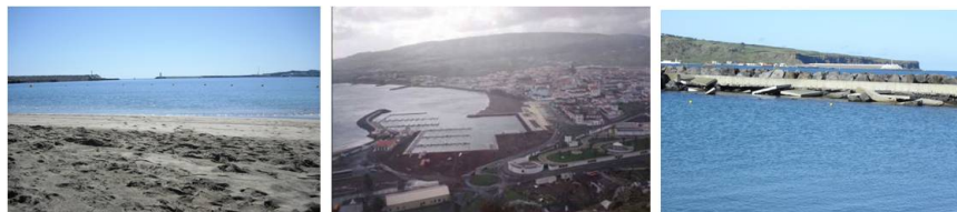
Figure 8: Coastal interventions inside Praia da Vitória bay (2 harbors, around 10 small jetties and a Marina) and identification of one damage jetty in 2009.
