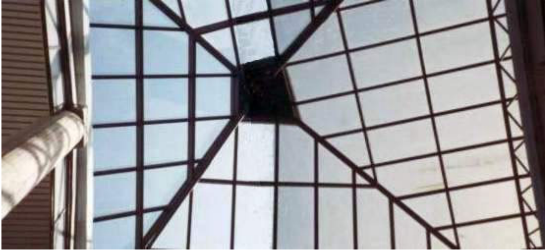
Photo 4: the new roof, invisible from the outside
